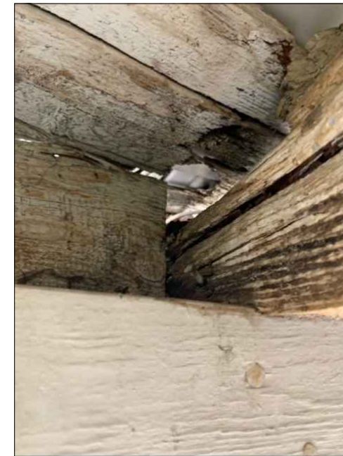
Existing Roof Framing Condition
