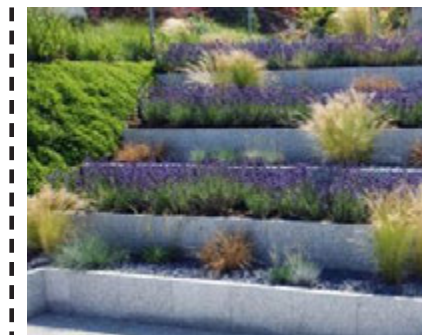
Cast-in-place concrete terraced retaining walls and planting
