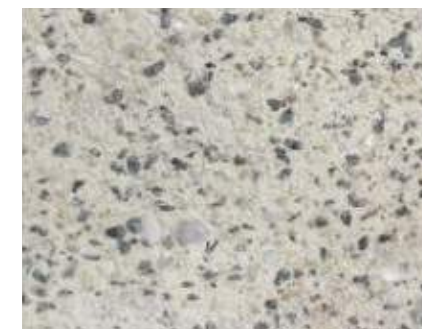
Sandblasted finish at cast-in-place concrete walls
