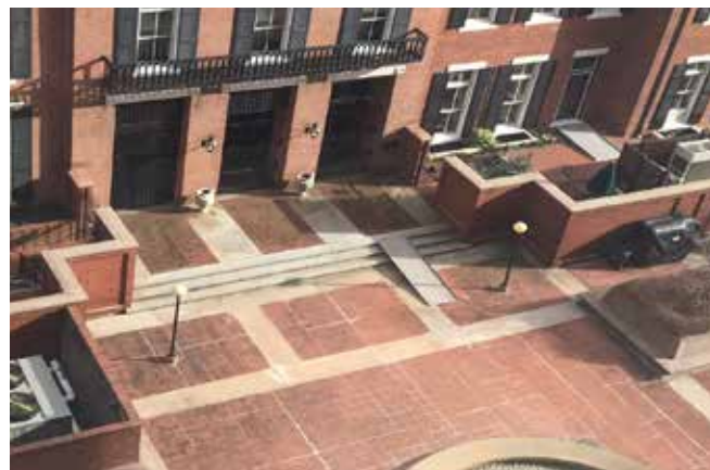
AERIAL VIEW OF EXISTING LANDING AND STEPS, TEMPORARY METAL RAMP TO BE REMOVED.
