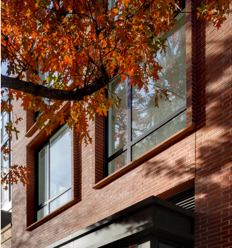
BRICK JAMBS + PRECAST SILL & LINTEL
