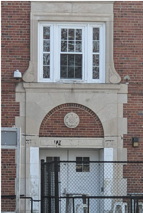
Historic Cast Stone on West Facade
