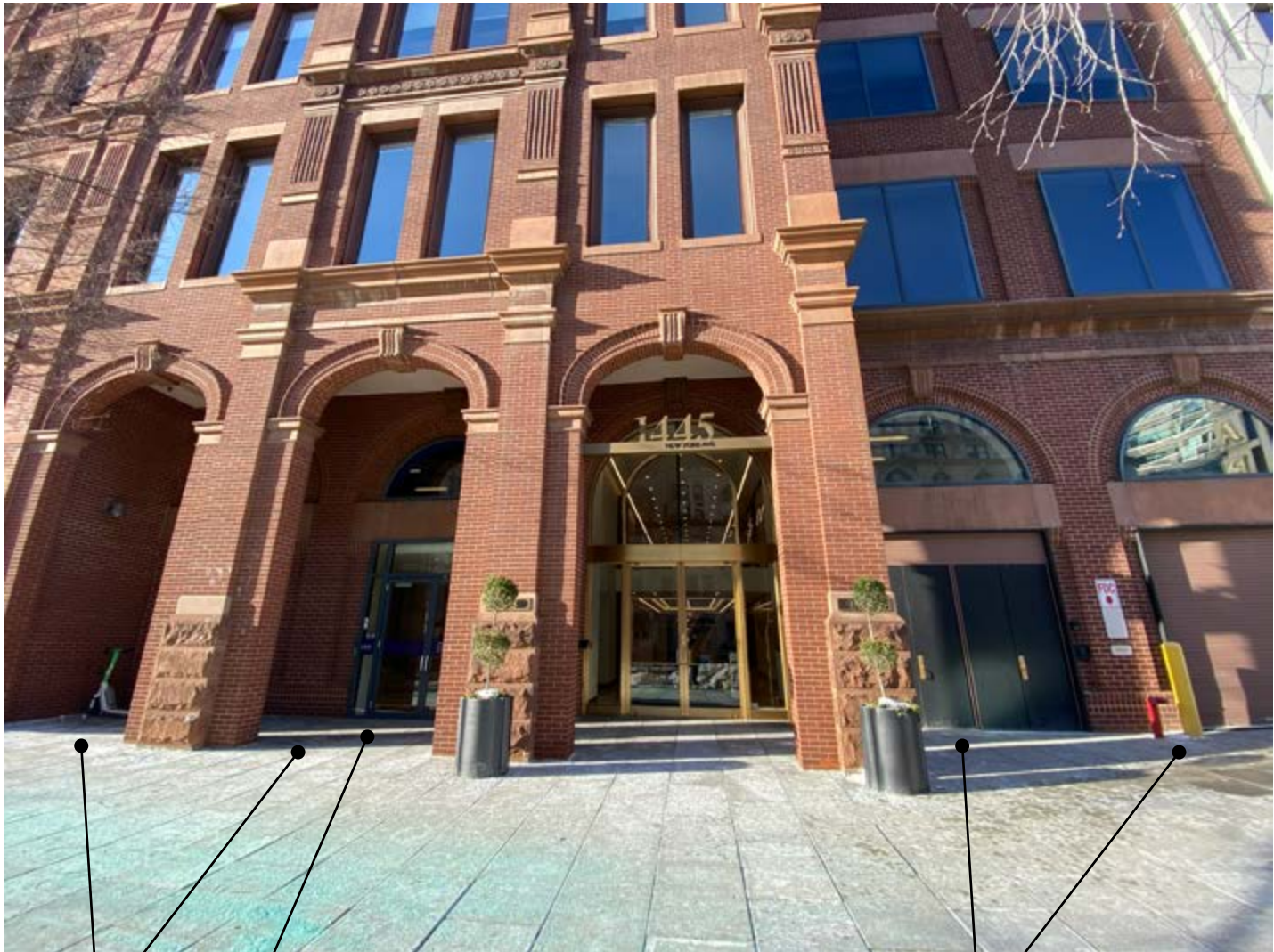
EXIT DISCHARGE DOORS AND OVERHEAD COILING LOADING DOCK ACCESS DOOR. THESE DO NOT CONTRIBUTE TO A GREAT FIRST IMPRESSION OF THE BUILDING.
