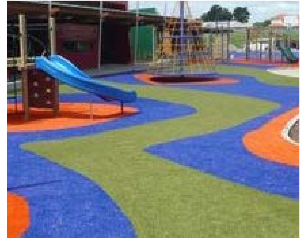
PERMEABLE P.I.P RUBBER SURFACE
