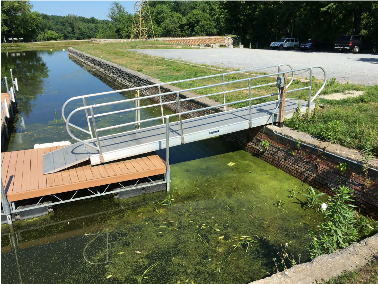
Figure 13: Example of the gangway design proposed for the project. This gangway, although shorter than that needed for Georgetown, is employed at multiple locations throughout the park.
