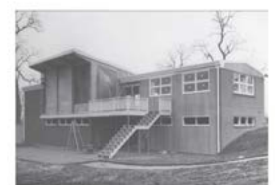
Existing Clubhouse under construction, 1964
