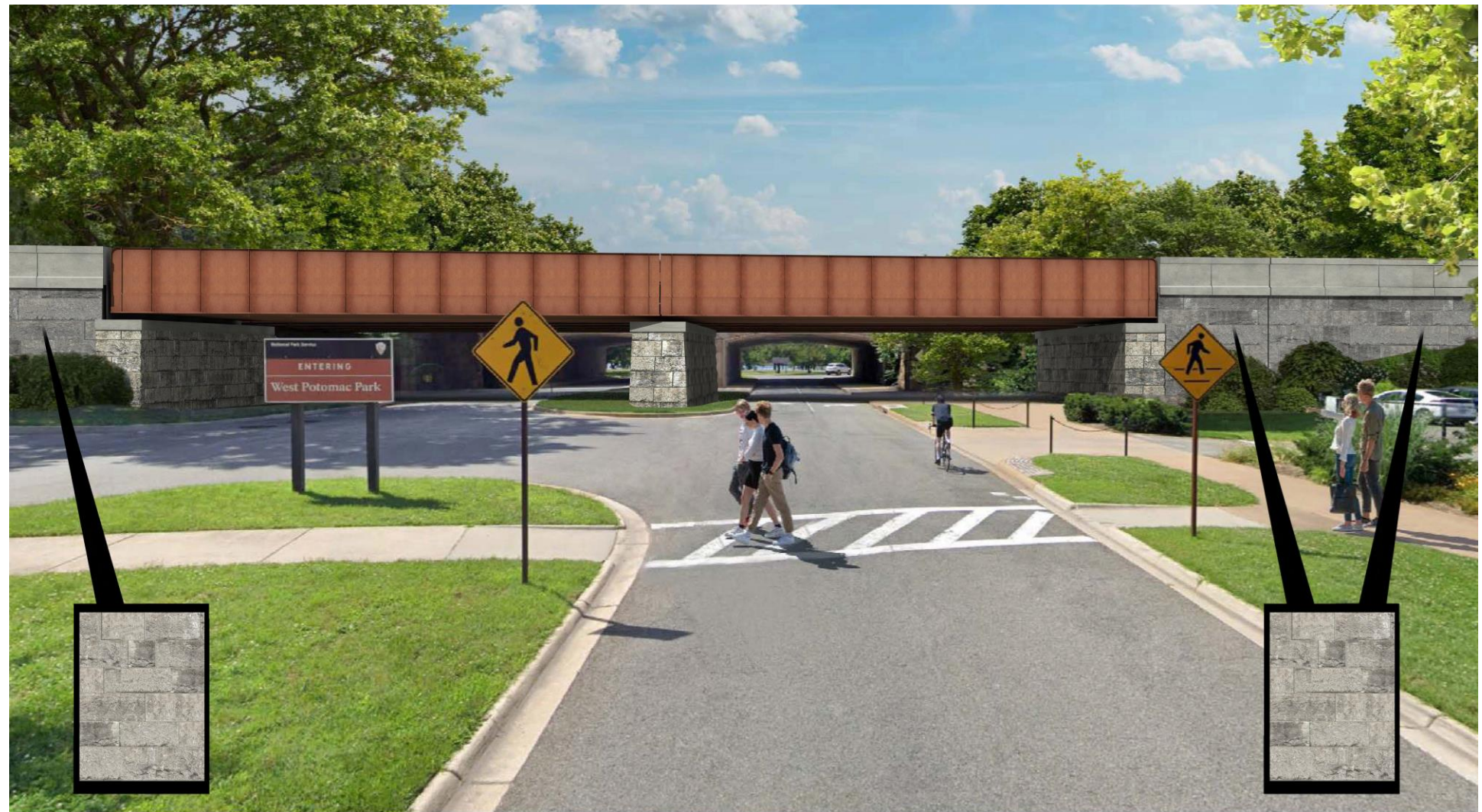
New Stone Cladding at Wingwall
