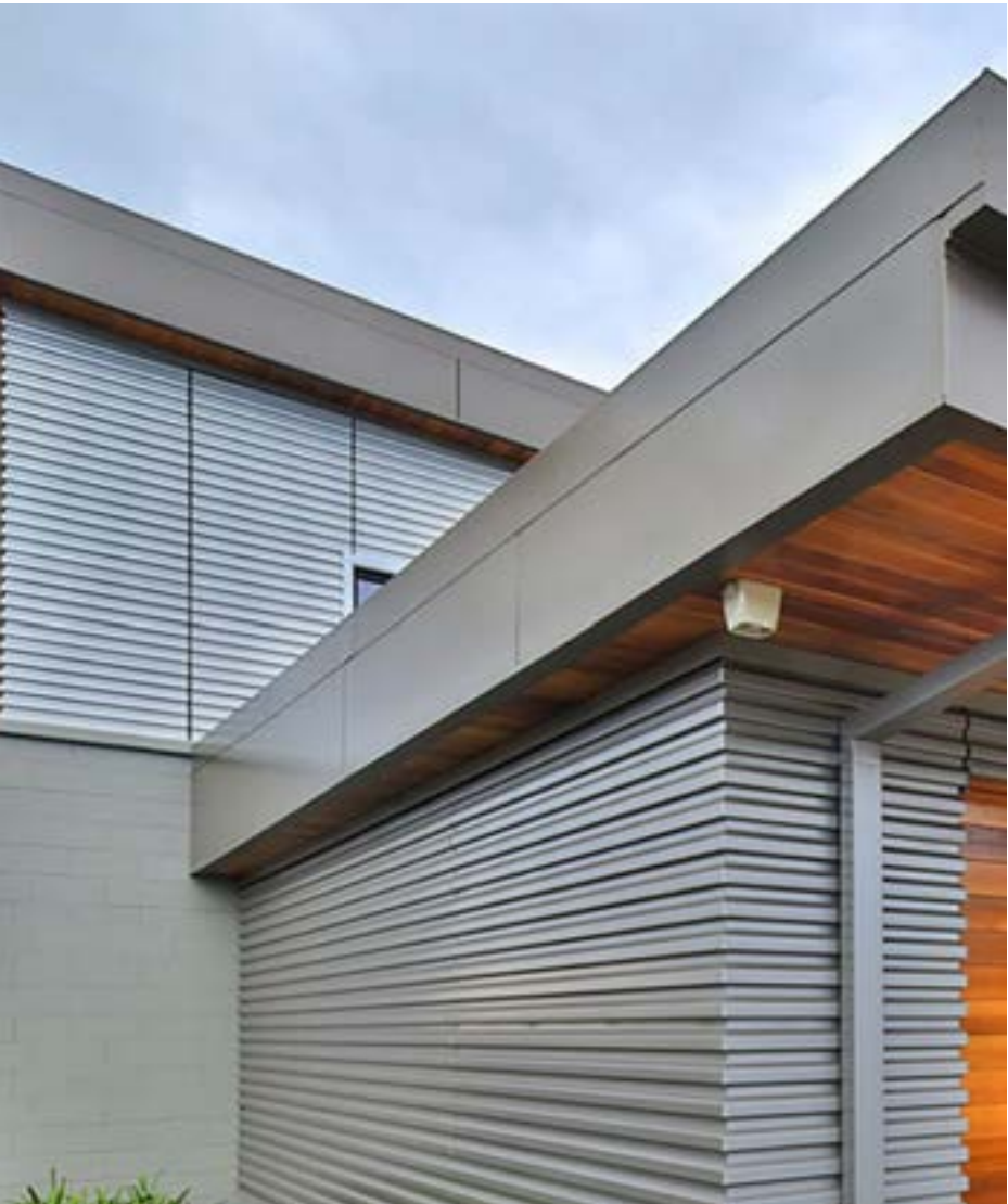
(Kingspan.us - DesignWall R-series - Proposed ribbed panel to be used in vertical orientation)
