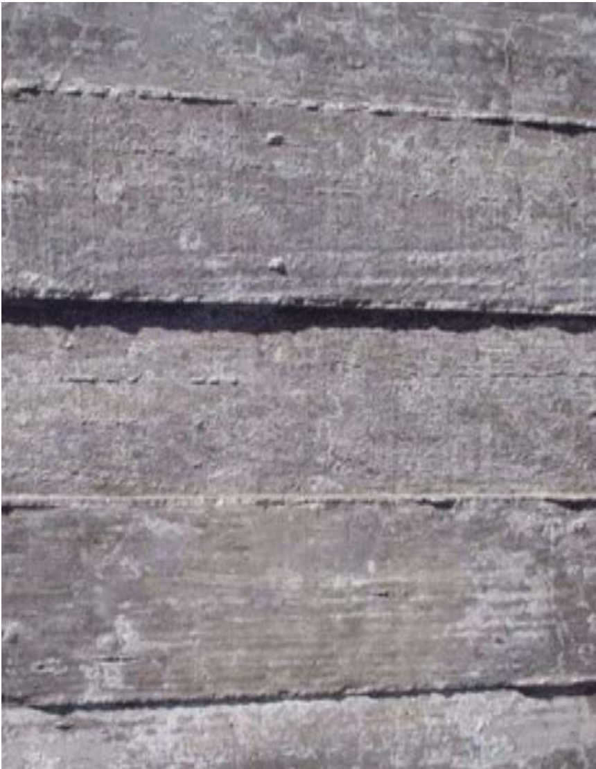
Detail of board-formed concrete at Hector Garcia Middle School, Dallas, TX, by Perkins&Will)
