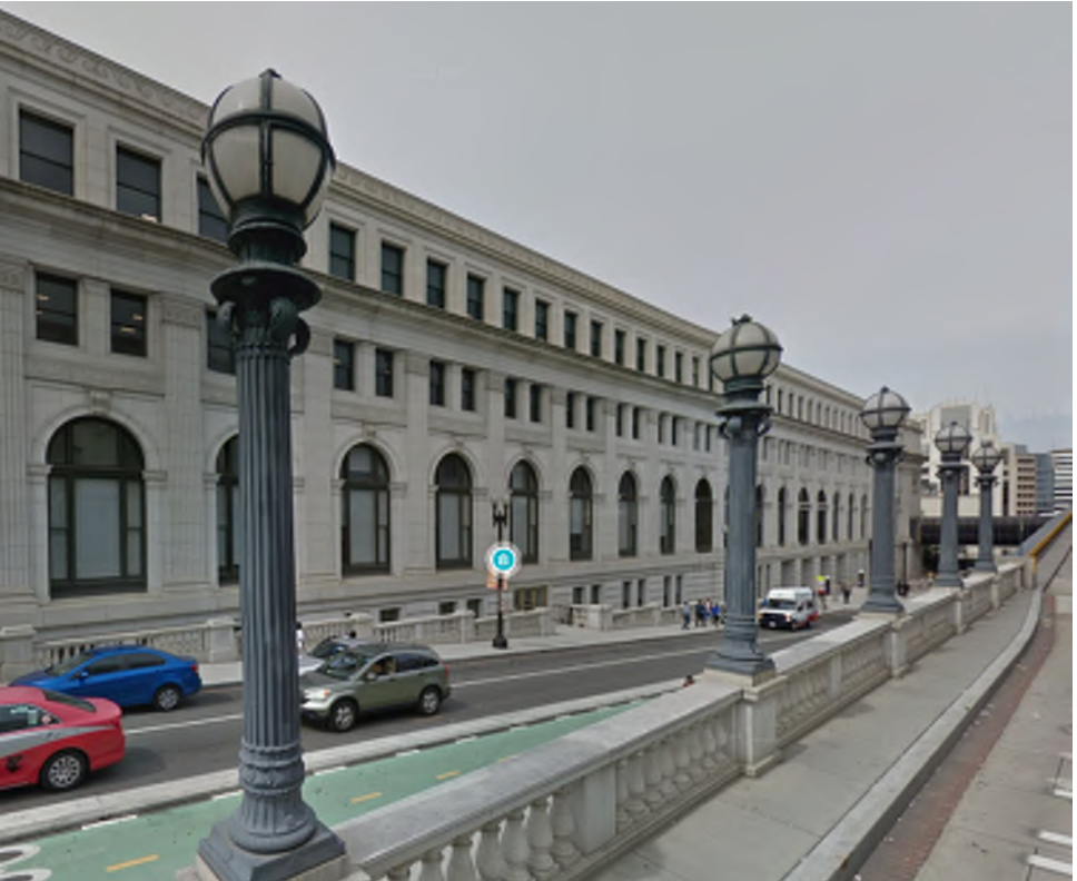
Rostral Lamp Posts along First Street
