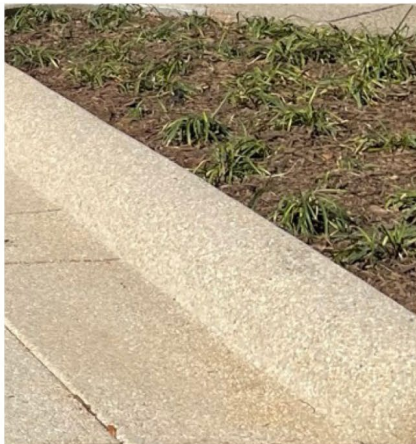
NPS Standard Quarter Round Curb, Exposed Aggregate Concrete
