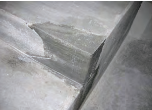
PATCHED CONCRETE STAIR
