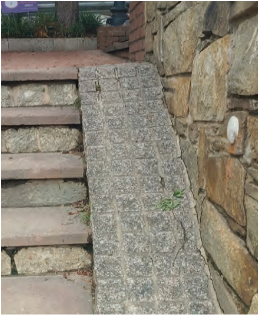
PAVED BIKE RAIL INTEGRATED INTO STAIRS AT C&O TRAIL
