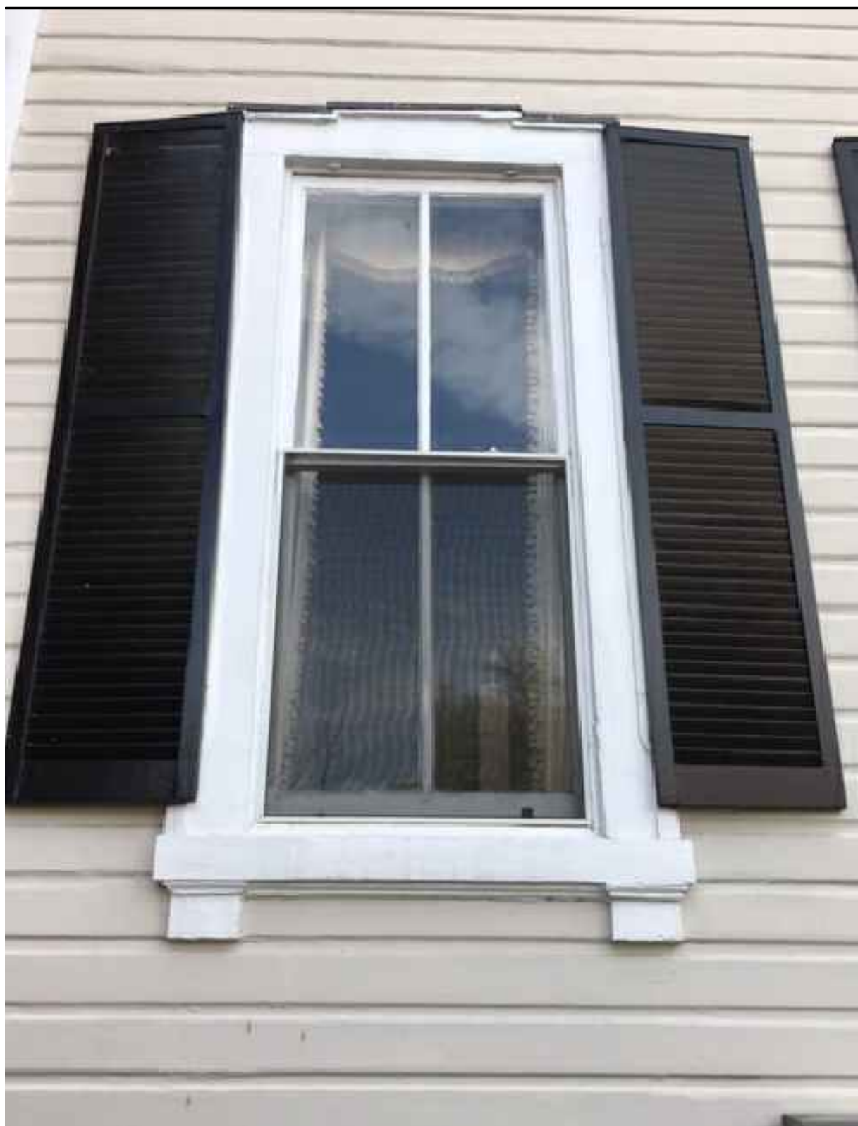
4 EXISTING EAST (FRONT) ELEVATION INOPERABLE LOUVERED SHUTTERS
