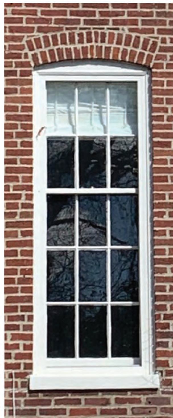
EXISTING FIRST FLOOR WINDOW
