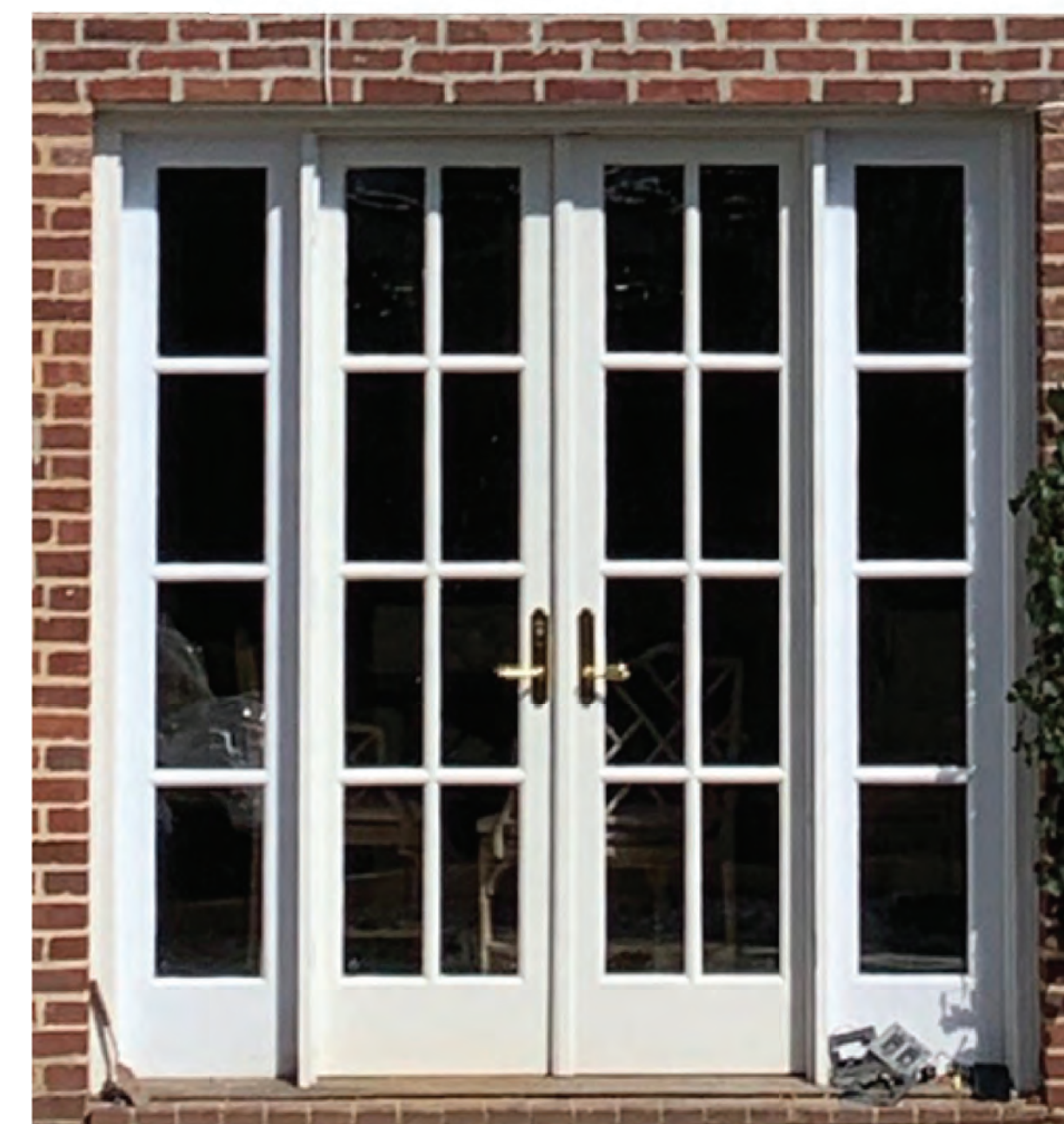
EXISTING BASEMENT DOORS
