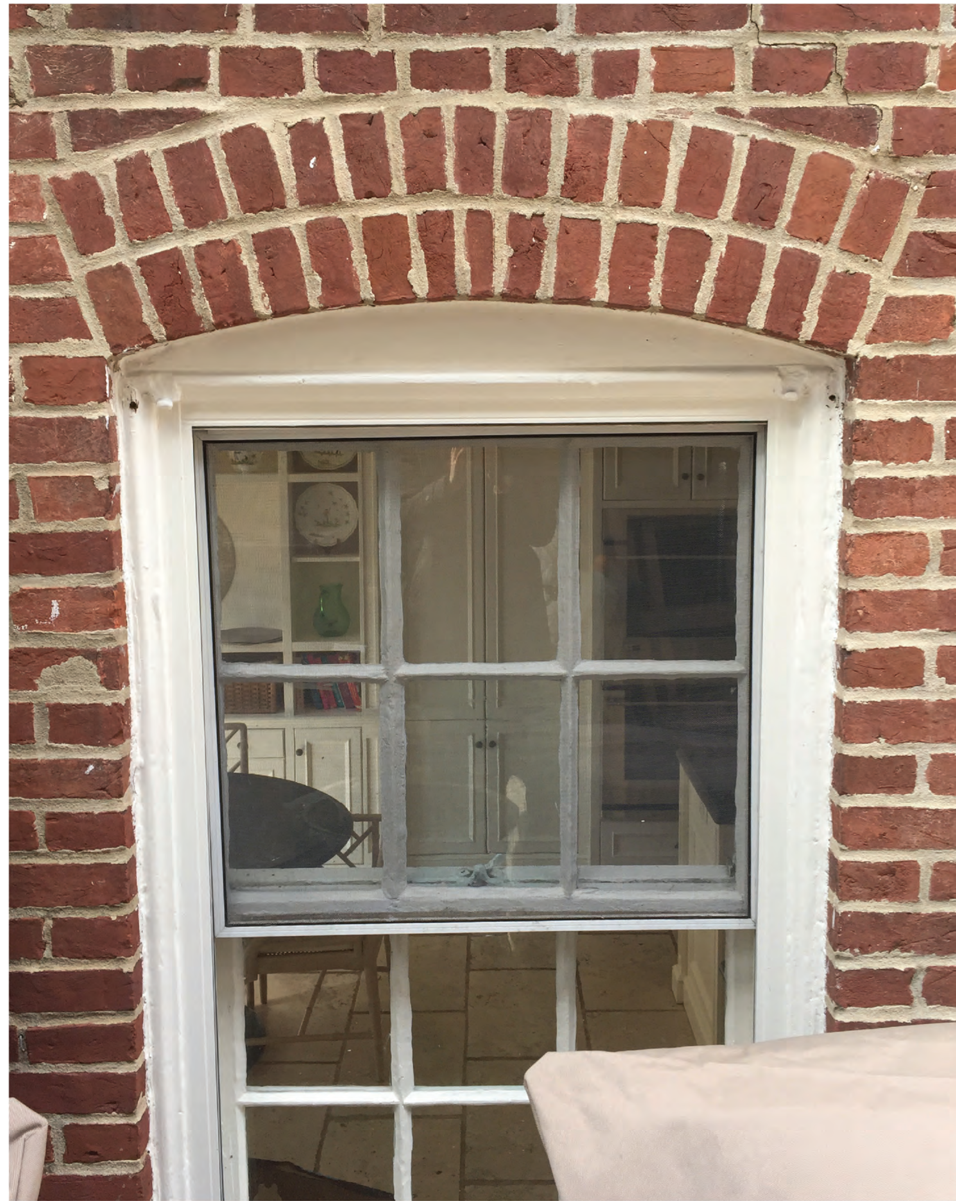
TYPICAL EXISTING WINDOW HEAD DETAIL
