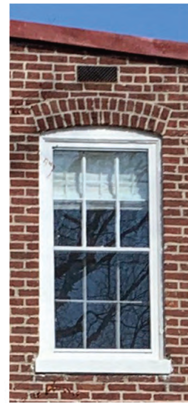
EXISTING FIRST FLOOR WINDOW
