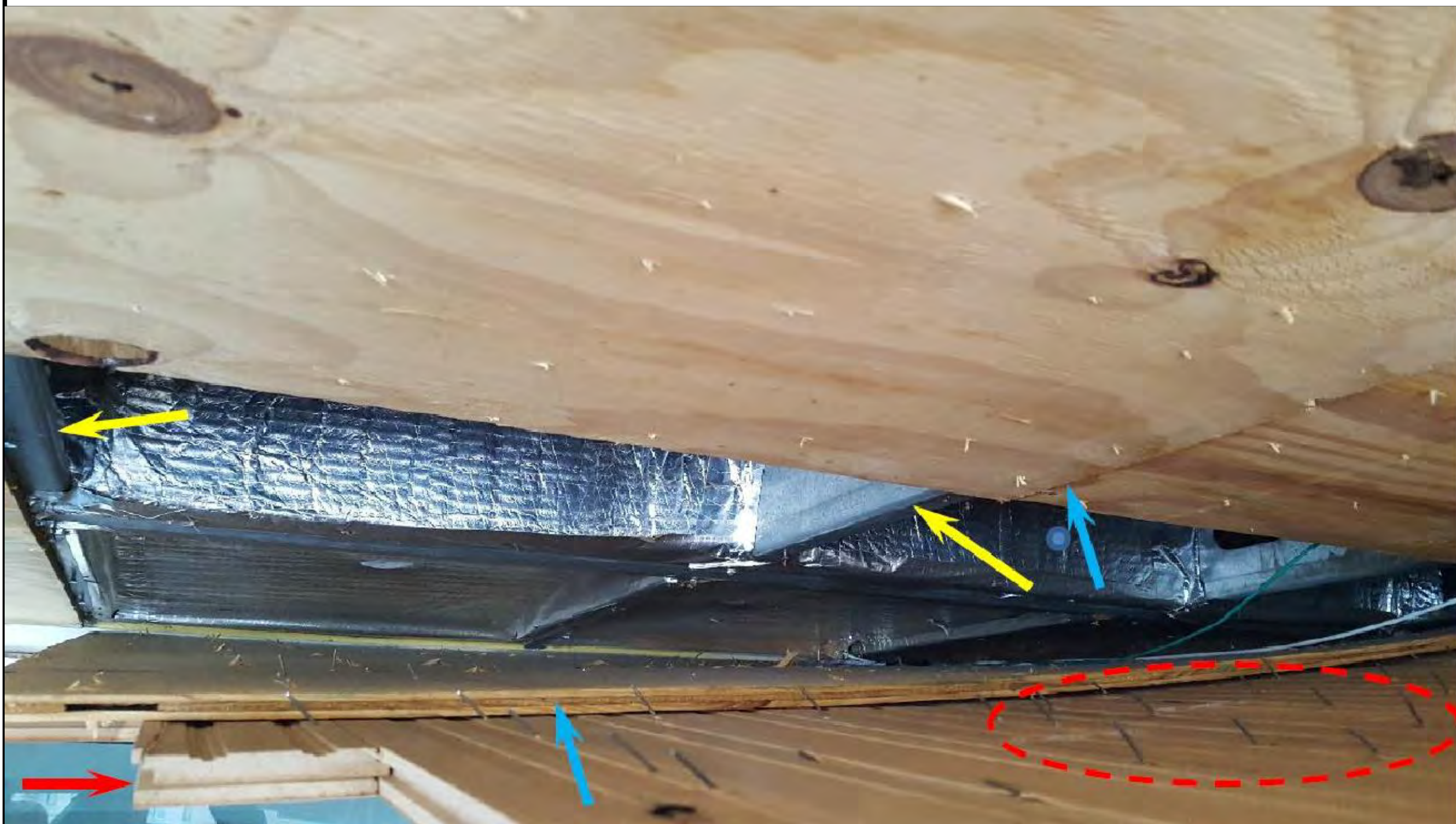
SOFFIT FINISH FALLEN AREA WEST SIDE
