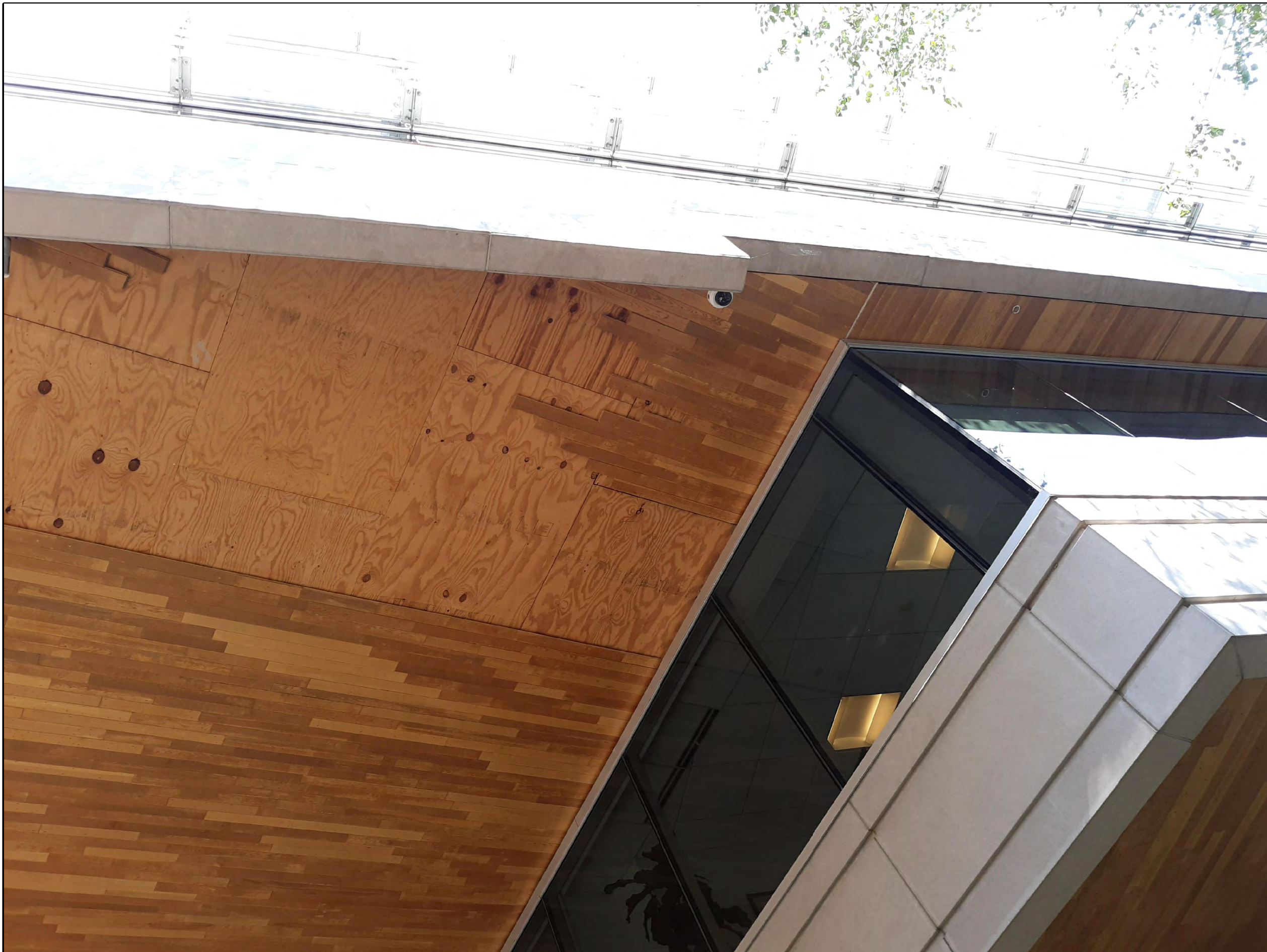
SOFFIT FINISH FALLEN AREA WEST SIDE
