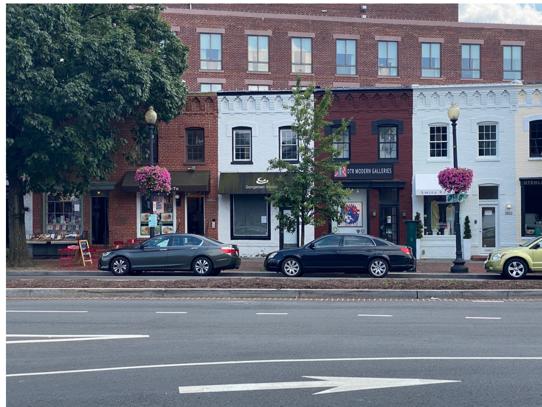
STREET FACADE (FROM ACROSS THE STREET)
