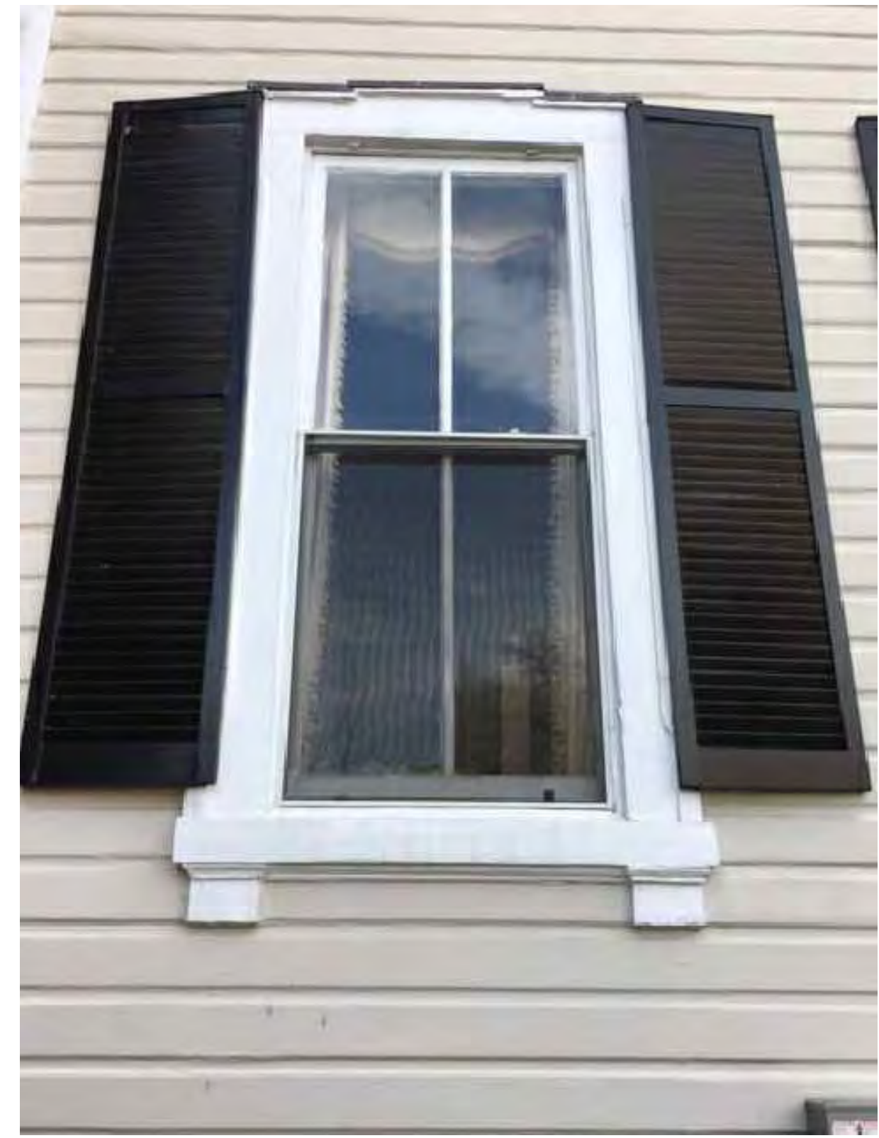
4 EXISTING EAST (FRONT) ELEVATION INOPERABLE LOUVERED SHUTTERS
