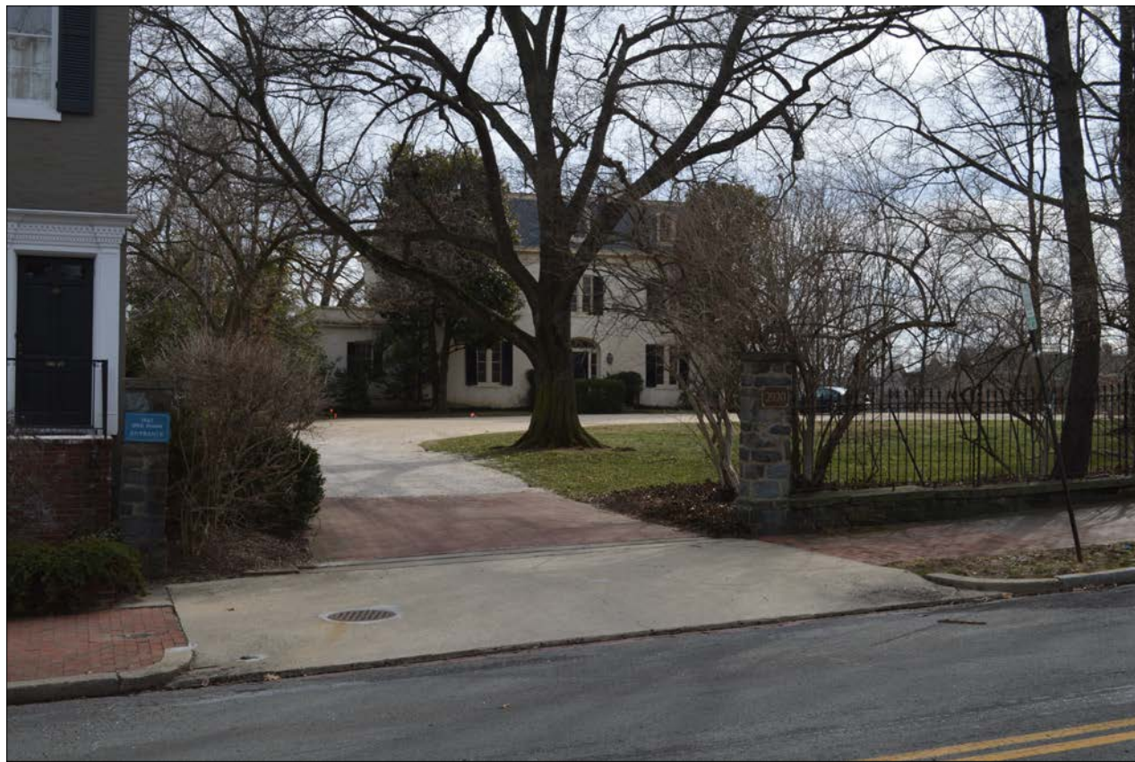
1 EXISTING VIEW FROM NORTH SIDE OF R ST. NW
