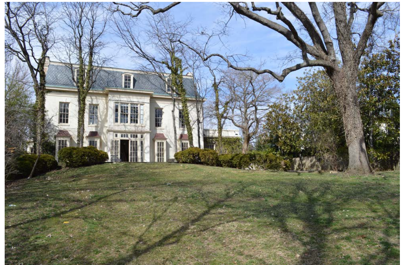
2 EXISTING VIEW OF SOUTH ELEVATION
