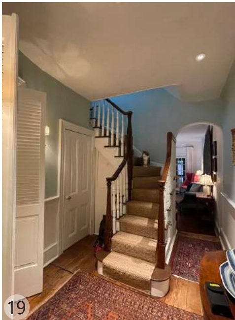
RESTORE LANDING AND LOWER STAIR RUN TO ORIGINAL CONFIGURATION USING HANDRAIL AND PICKETS SALVAGED FROM SOUTH STAIR TO BE REMOVED
