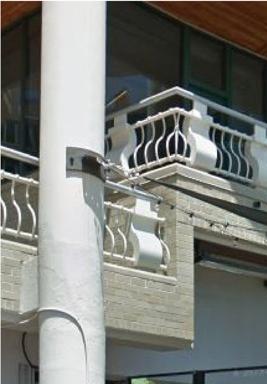
Washington Harbor Column w/ current canopy connection
