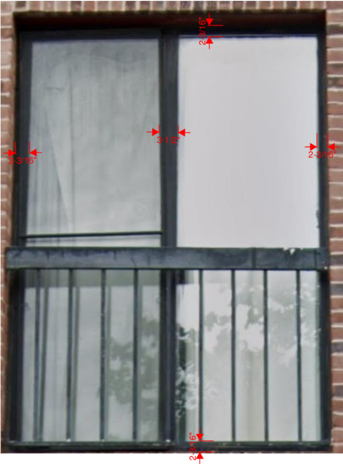
Closeup Exterior Photo (Glass is in the same plane on both windows and is not a sliding door):
