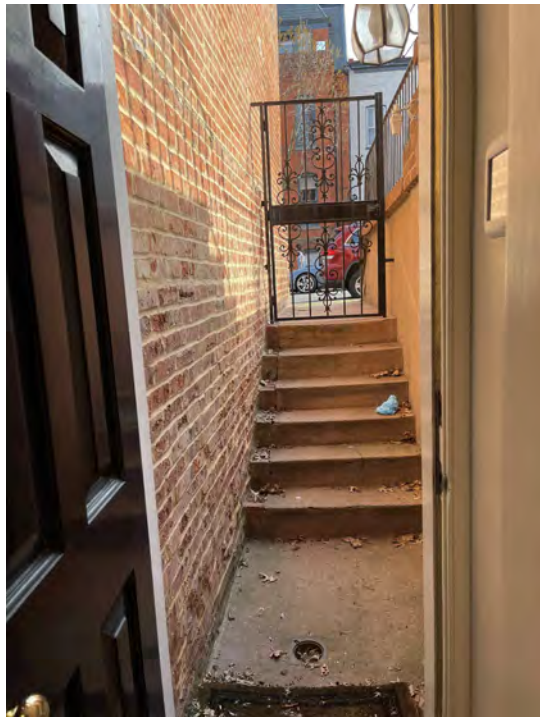
C4 9 EXISTING STEPS TO LOWER LEVEL DOOR
