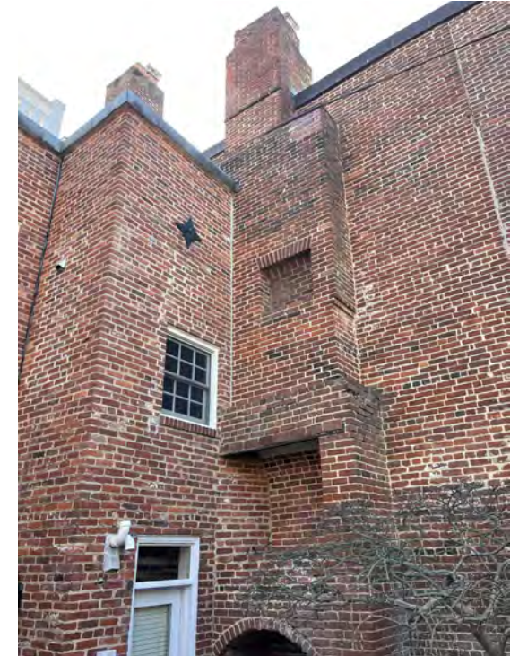
A4 EXISTING BRICK CHIMNEY VIEW 10 NA
