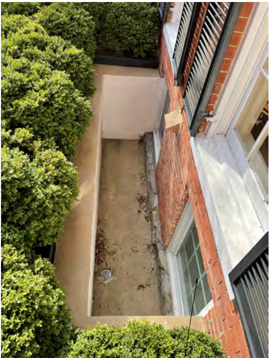
C2 9 EXISTING WINDOW WELL AT FRONT ELEVATION
