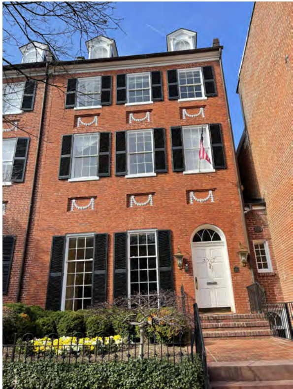
A1 9 FRONT VIEW OF PROPERTY
