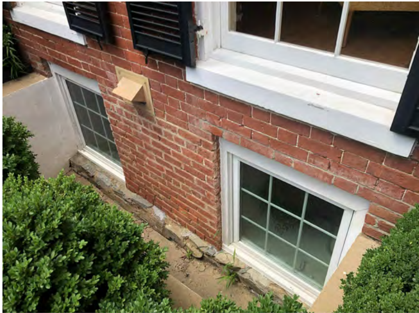
C1 9 EXISTING WINDOW WELL AT FRONT ELEVATION
