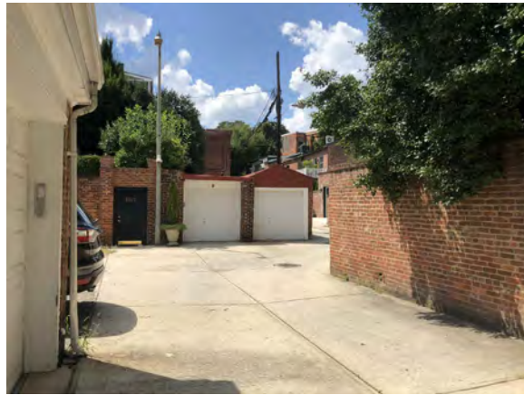
A4 || EXISTING REAR (ATTACHED) GARAGE VIEW NA
