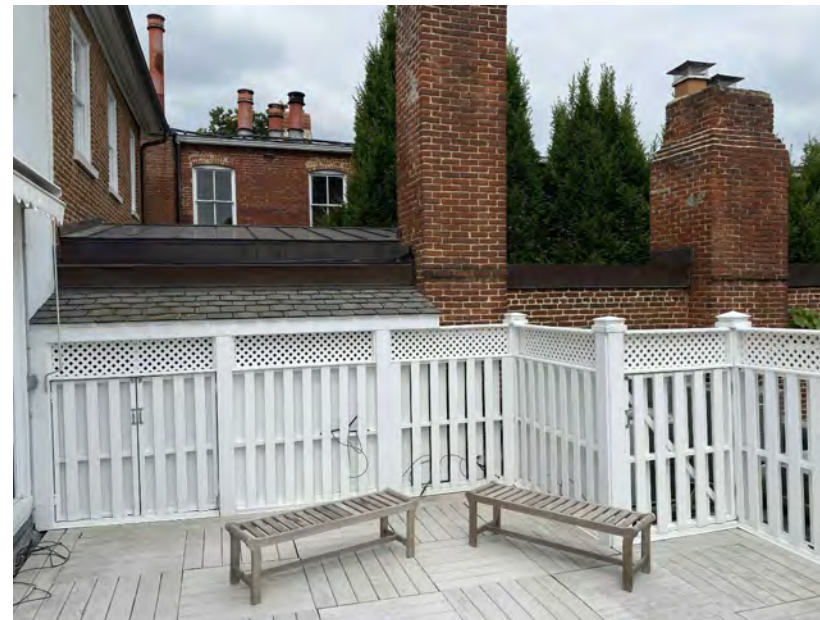
C2 EXISTING SECOND FLOOR DECK VIEW 10 NA
