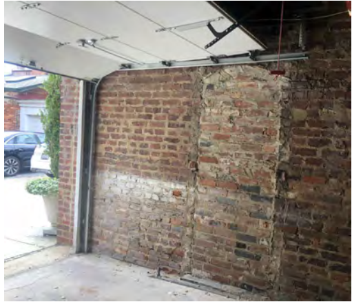
A1 || EXISTING REAR (ATTACHED) GARAGE VIEW NA
