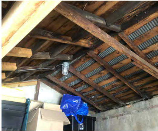
A2 || EXISTING REAR (ATTACHED) GARAGE VIEW NA
