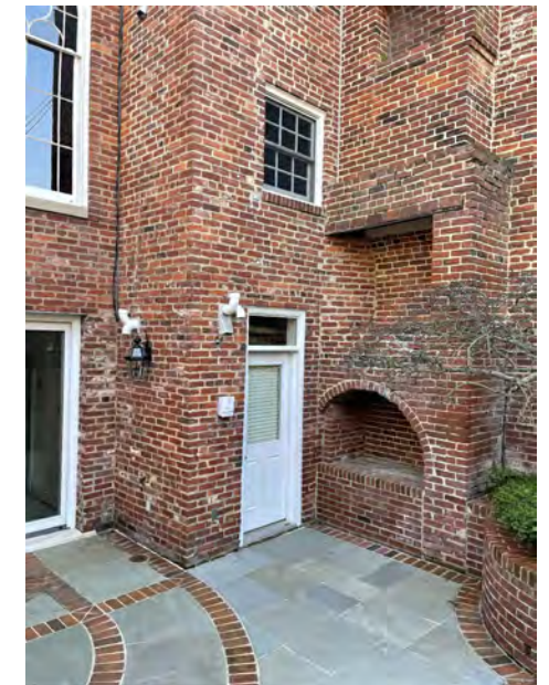
C4 EXISTING BRICK CHIMNEY VIEW 10 NA
