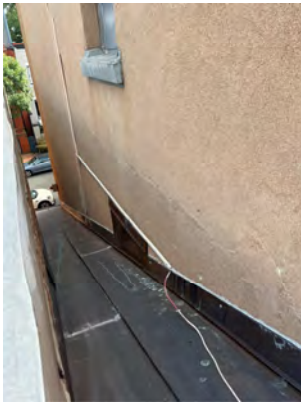
A2 14 EXISTING EAST SIDE ROOF NA
