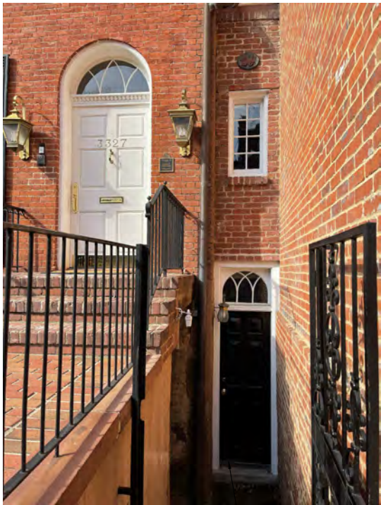
C3 9 EXISTING LOWER LEVEL DOOR VIEW
