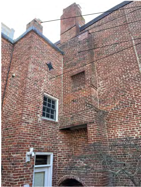
A3 15 EXISTING BRICK CHIMNEY VIEW NA REPOINT CHIMNEY AND WALL
