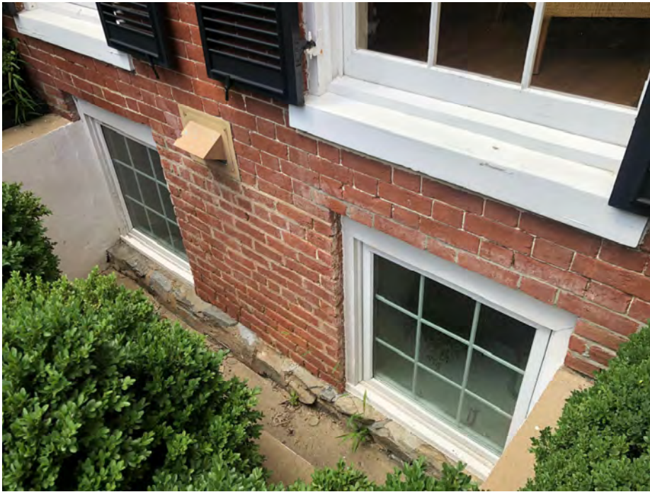
C1 13 EXISTING WINDOW WELL AT FRONT ELEVATION TO BE REPLACED NA
