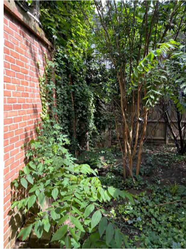
3. EXISTING MASONRY WALL TO REMAIN
