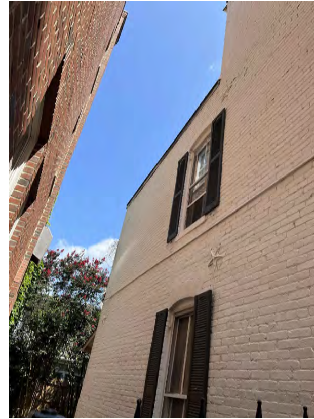
4. REAR EXISTING ADDITION
