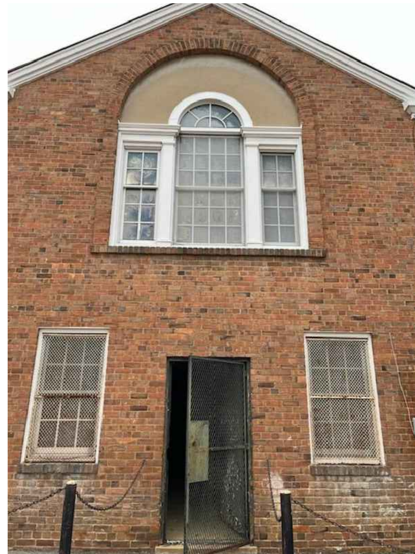
5 PAVILION EXISTING REAR- VIEW 03 NTS
