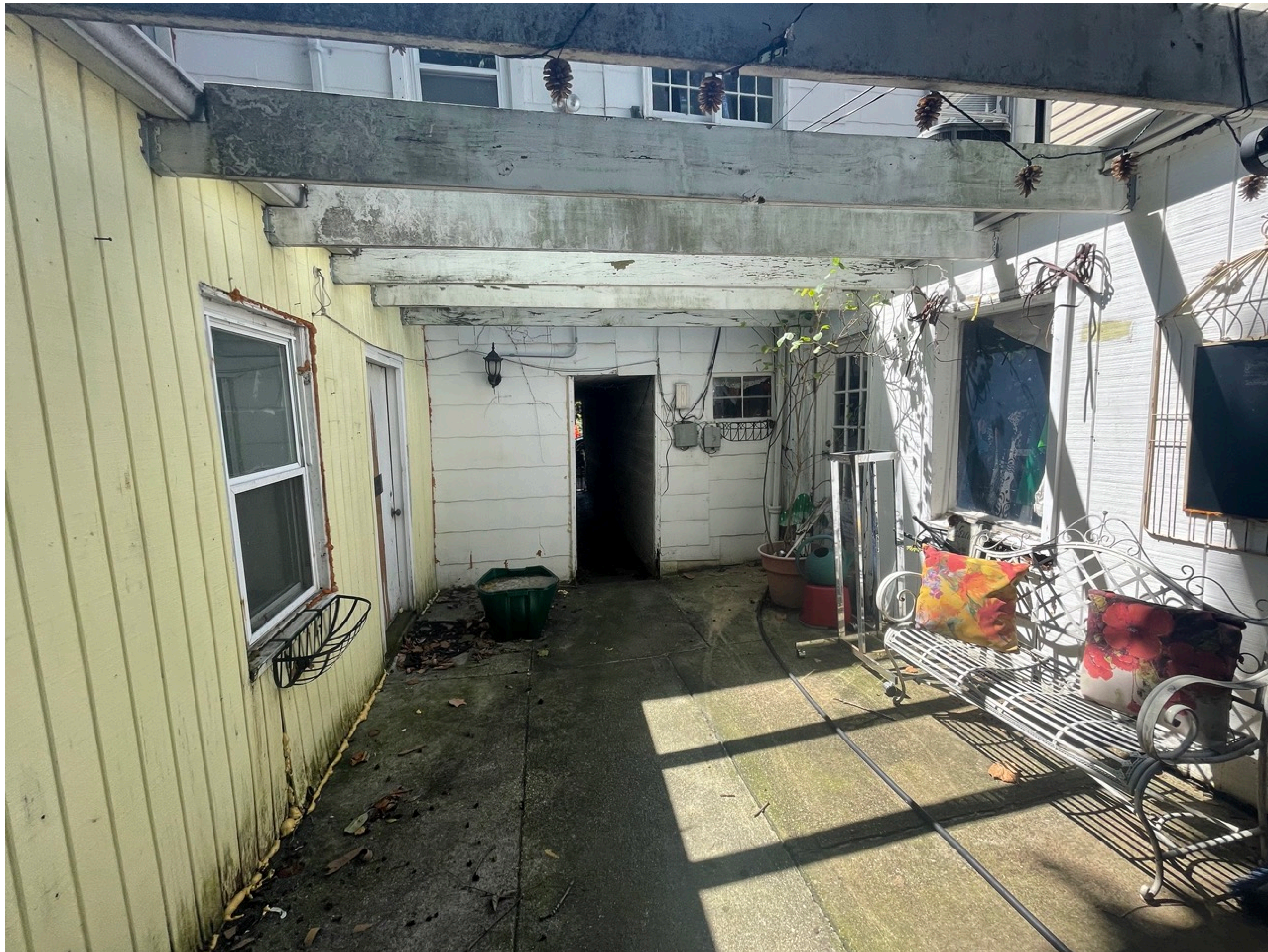
EXISTING REAR YARD
