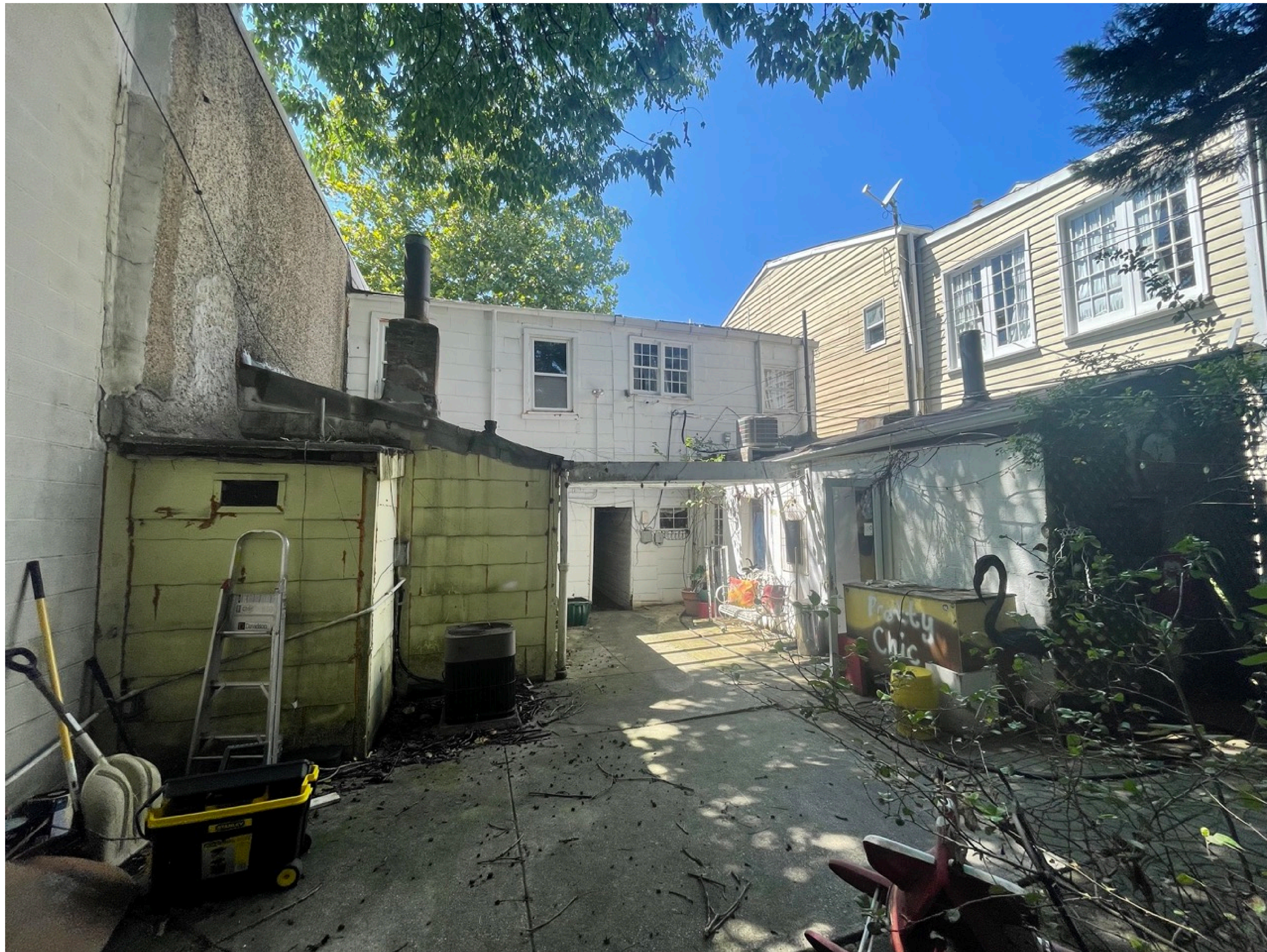
EXISTING REAR YARD
