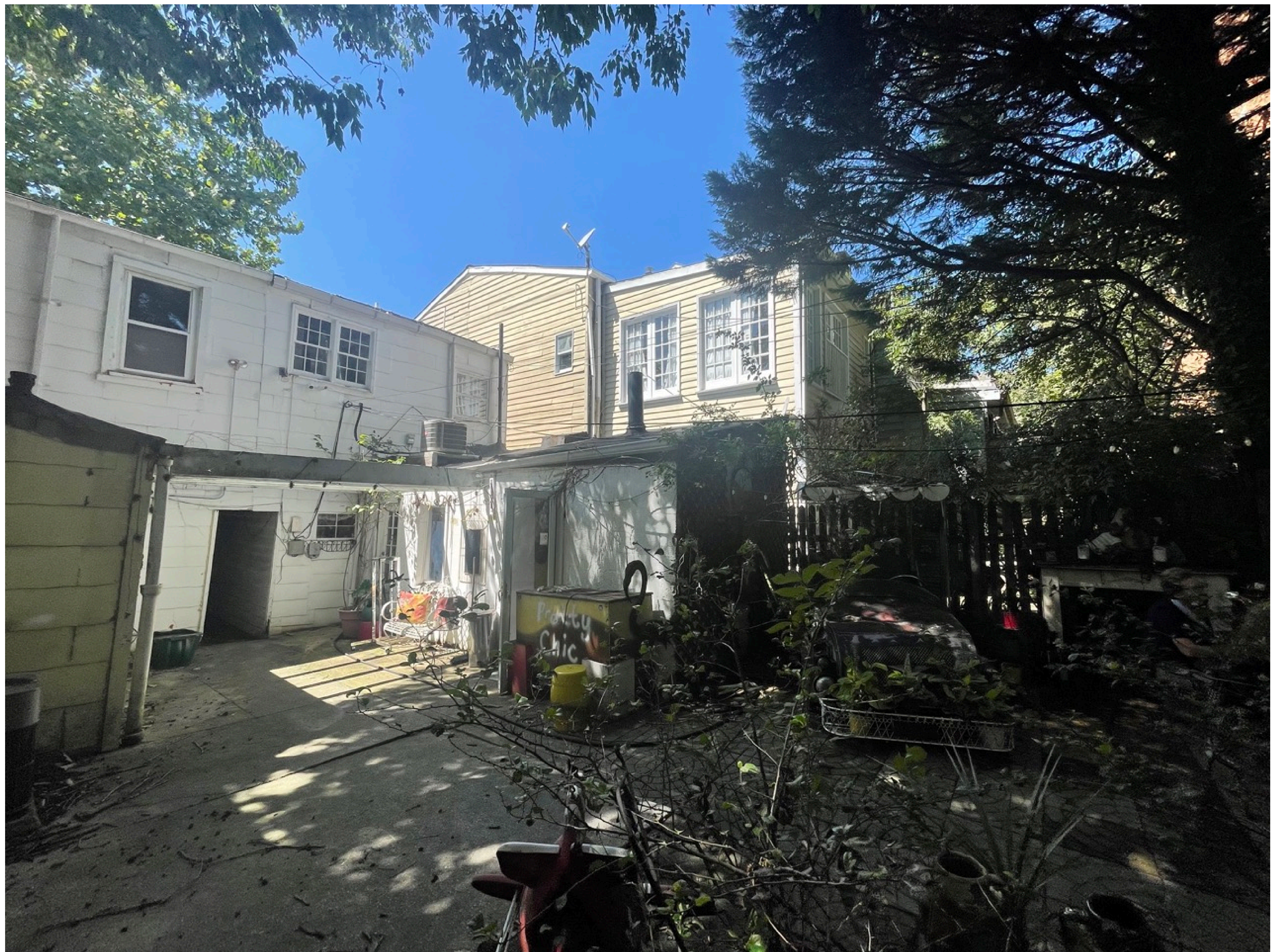
EXISTING REAR YARD
