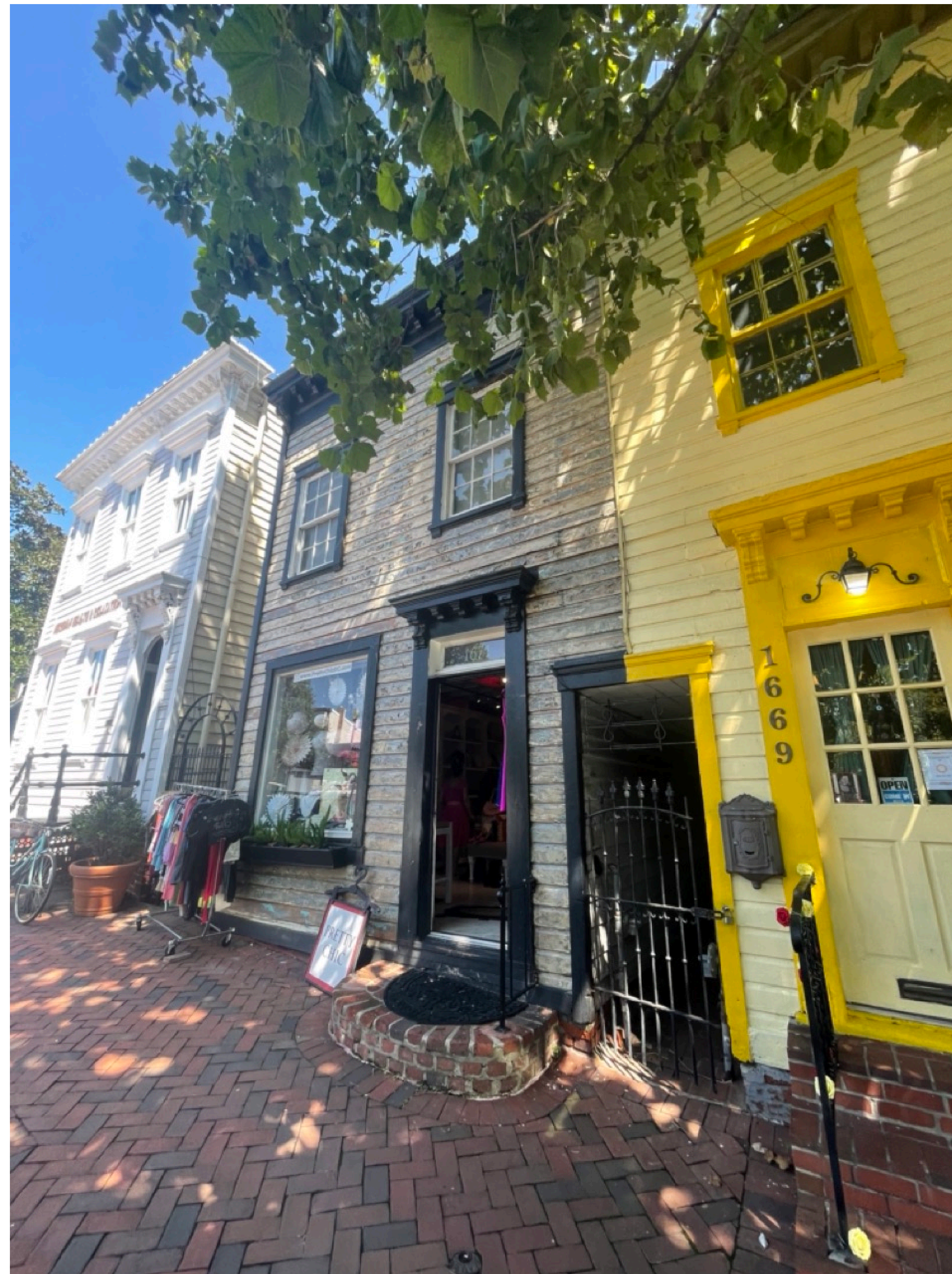
EXISTING FRONT FACADE
