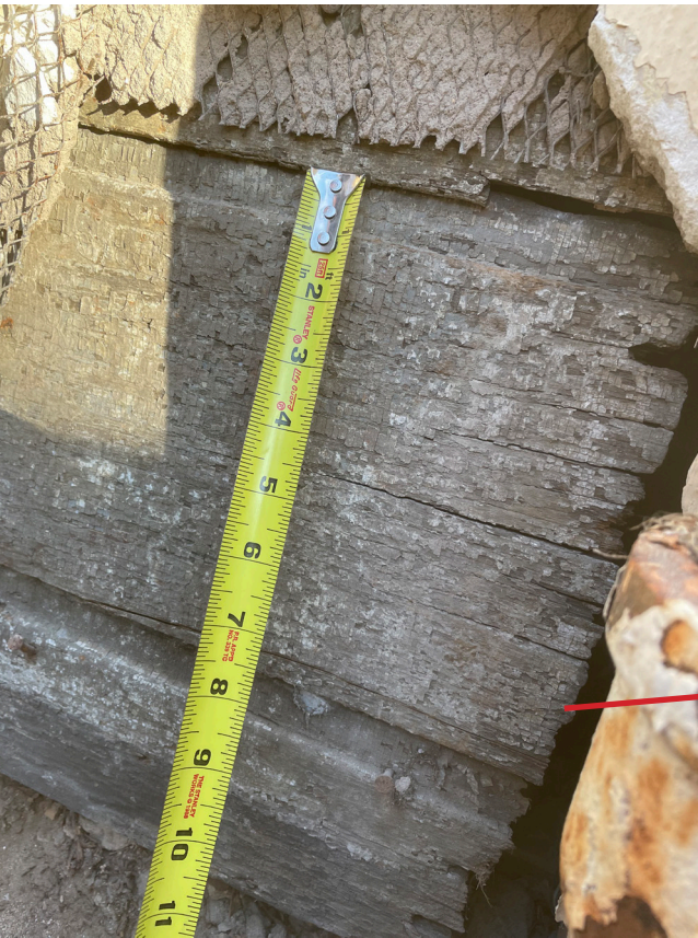
Image of 8" shiplap siding beneath existing stucco
