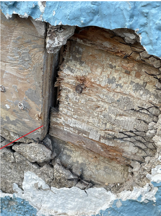
Photograph showing existing siding beneath plaster and lath on front elevation showing 6" german profile siding
