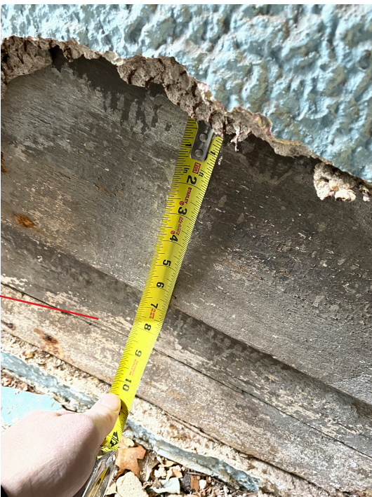
Photograph showing existing 6.5" lap siding beneath plaster and lath along the wall in the arched alley
