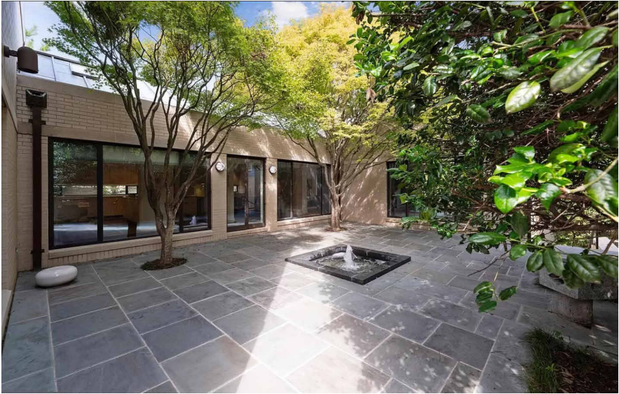
Existing East Elevation in Courtyard
