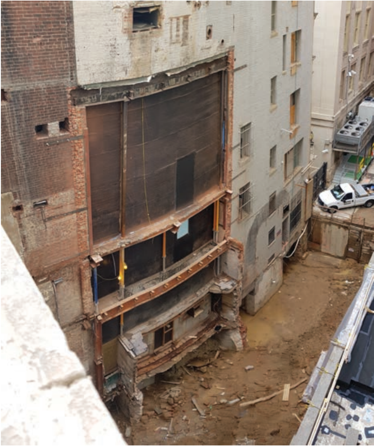
C. DEMOLITION OF 1503 NORTH BAY AND FACADE
