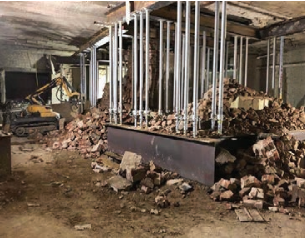
L. SHORING AND EXCAVATION OF 1501 L1
