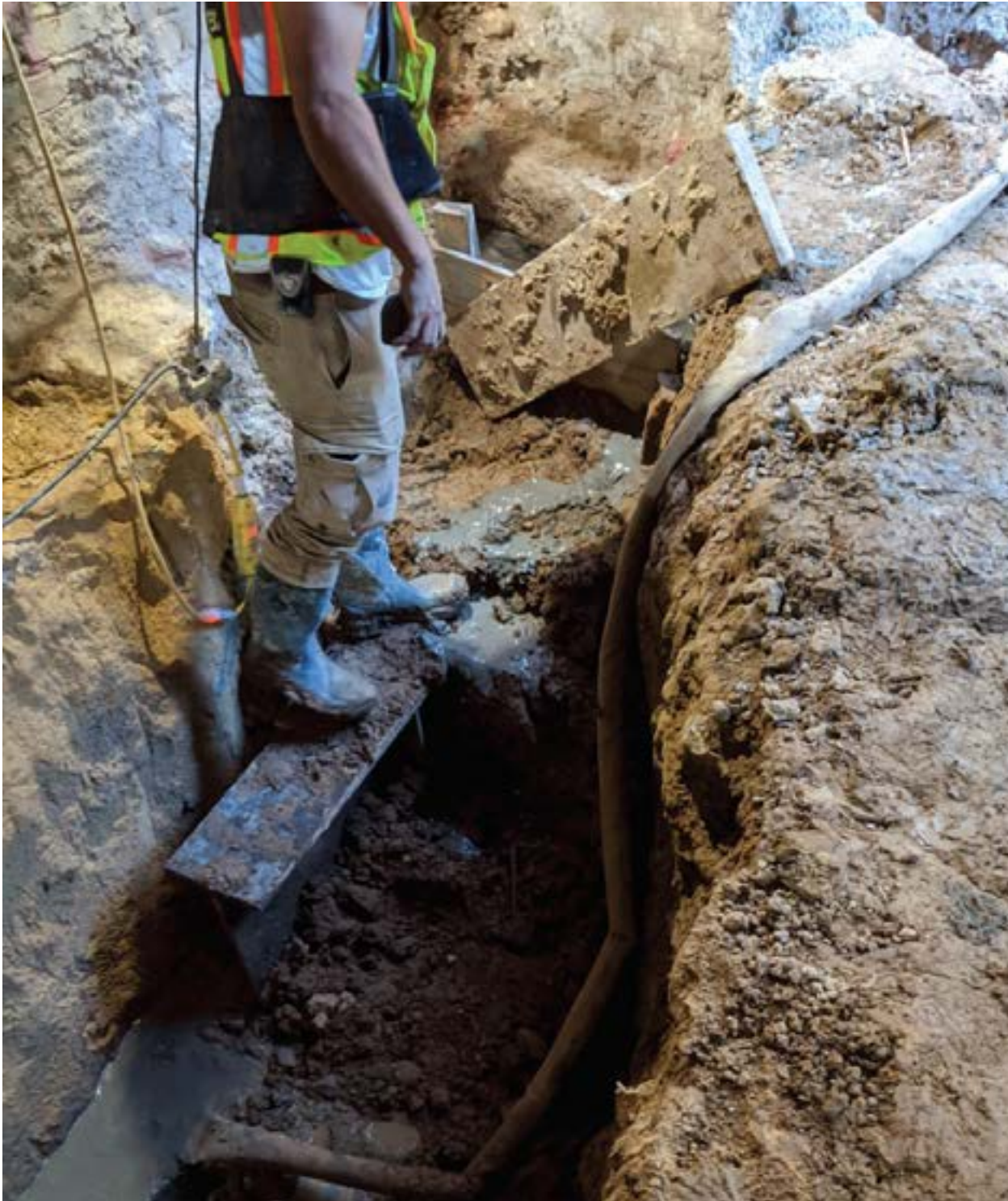
E. COMPLETION OF NEEDLE BEAM BELOW 1505 FOOTING
