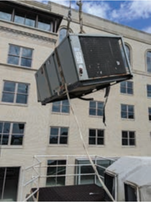
D. DEMOLITION OF 1505 ROOFTOP EQUIPMENT
