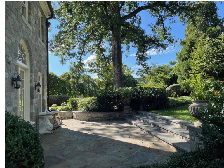
3. North Elevation Side Close-Up
