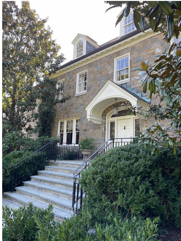
1. Front Entrance or East Elevation
