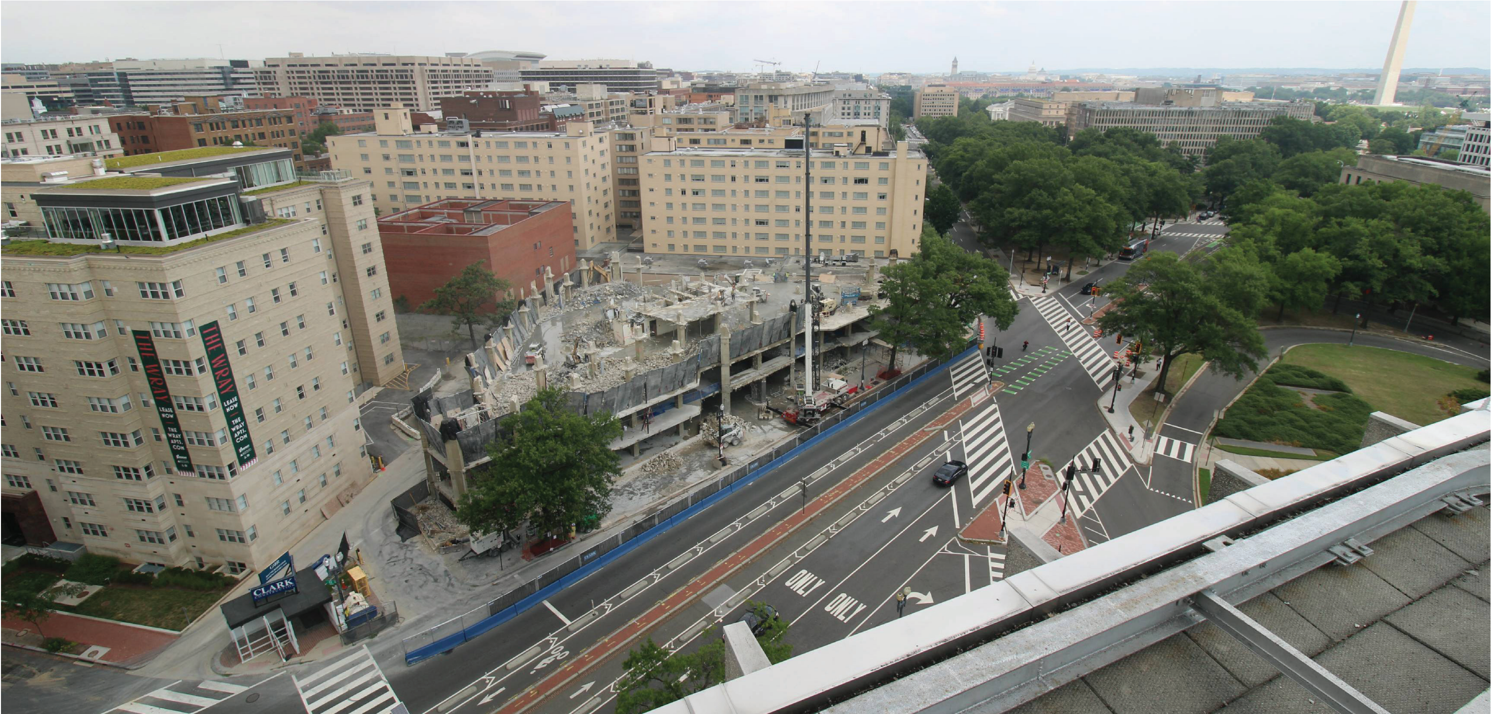
Existing above grade structure is currently under demolition under DOB Permit No. D2600067.
